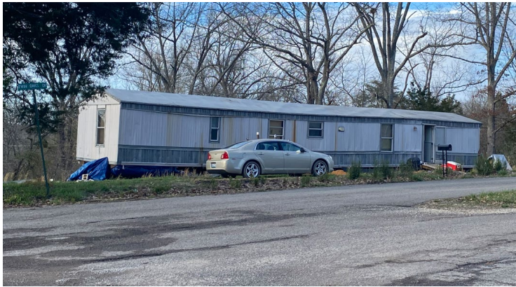
14'x70' Manufactured Home (1988) On site since March 2024
