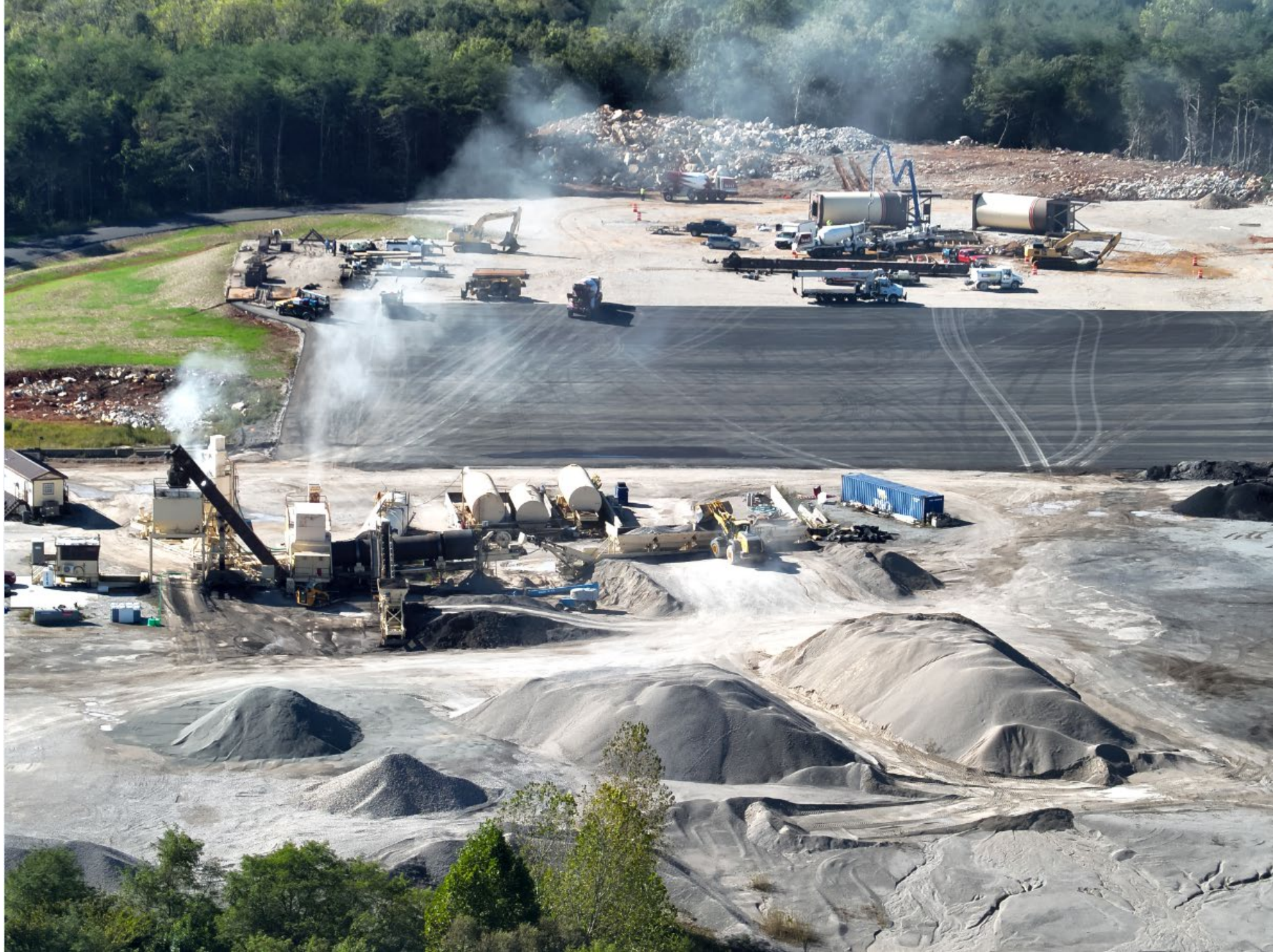
Existing Scotty's plant and site of future plant under construction
